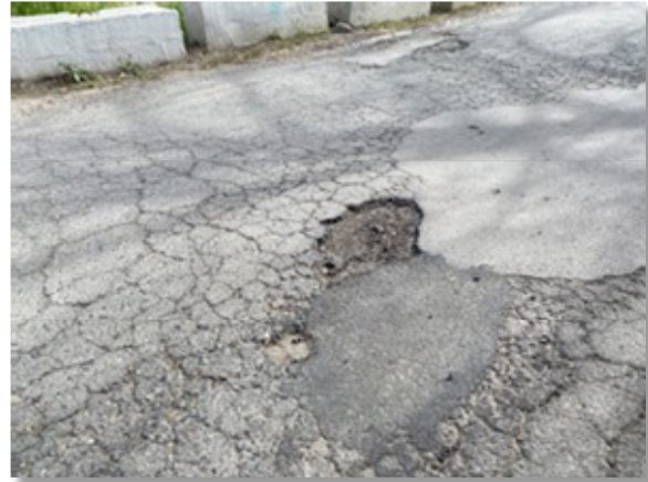
Parking lot condition.
