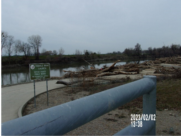
Debris from rising waters.
