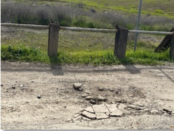
Road conditions inside facility.
