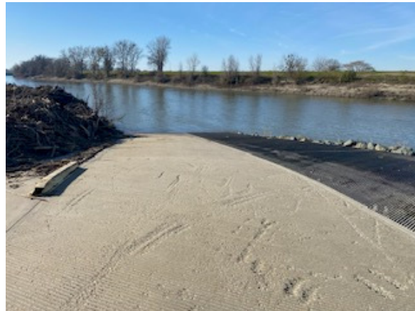
Launch with no floating dock.
