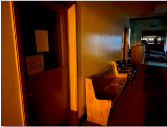
North wing looking South.
