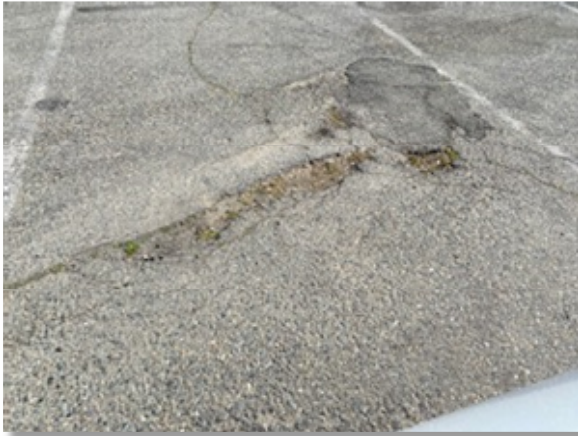
Parking lot condition.
