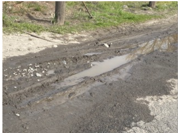
Road conditions inside facility.
